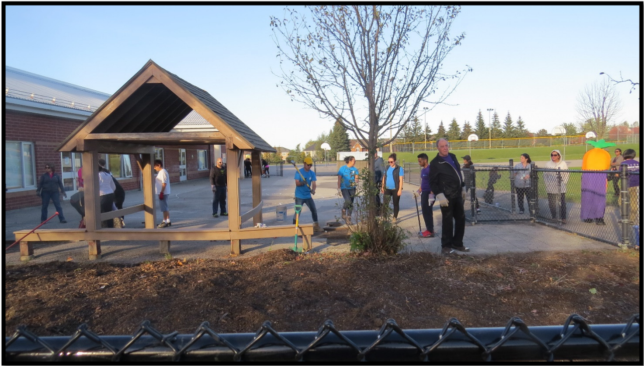
The workers pulling up pavement.
